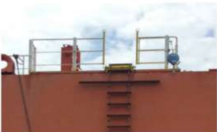
Figure 2: Gap in handholds appear to accommodate spreader.
